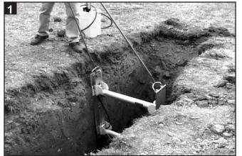
To remove the shore, place the removal tool through the handle with the hook facing the trench. Place the end of the tool over the same fitting where hose was hooked.
