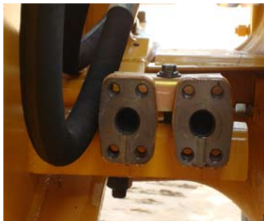
Fig.2 Original fitting removed
