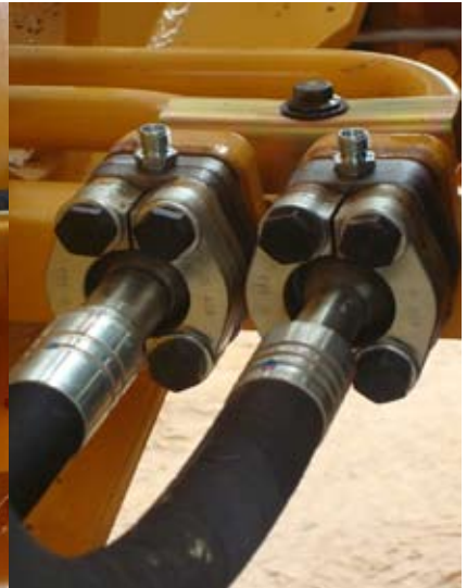
Fig.5 Fitting install completed
