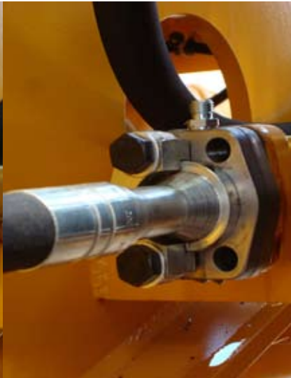
Fig.4 Original fitting and pipe back in place
