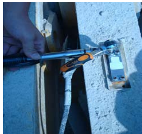
Fig.3 Load Link fitting
