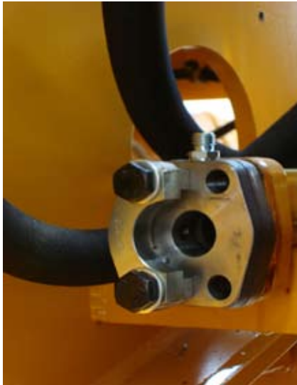
Fig.3 Vei flange fitting install
