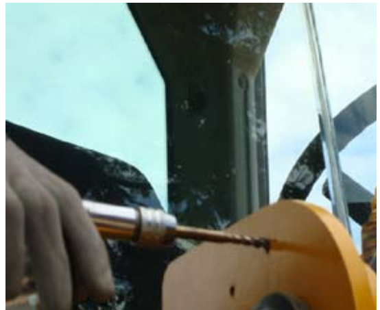
Fig.4 Tapping Weighing Zone bracket fixing points
